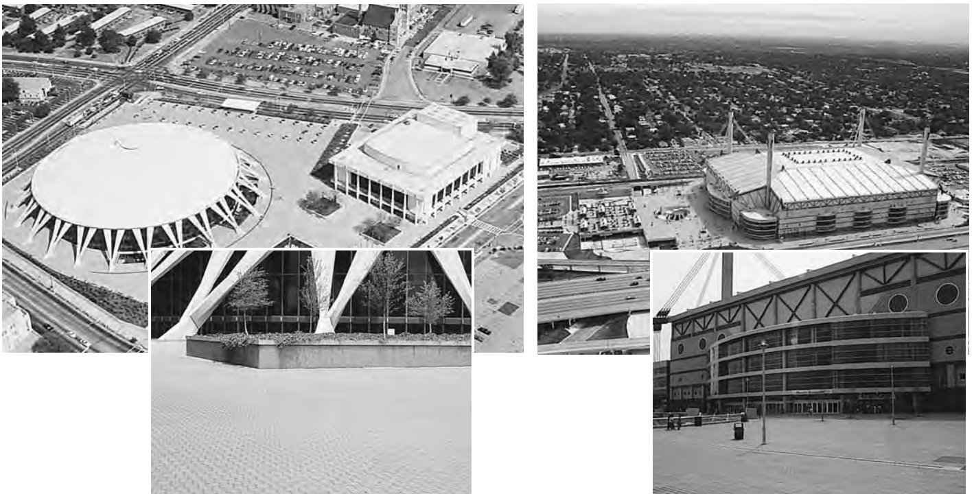
Figure 21. The plaza area around Scope Center in Norfolk, Virginia, (left) and one side of the Alamo Dome (right) in San Antonio, Texas, include roof plaza decks surfaced with concrete pavers.
