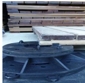
Ipenema on PCI Titan on PCI Hercules (note pins and slope correctors)
